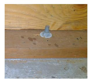
A home that is not properly bolted to its foundation could slide off of it during a CSZ earthquake, making it unsafe for occupation
